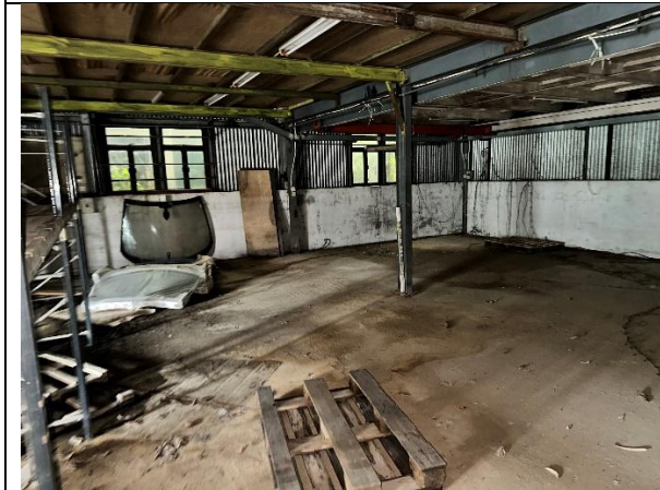
11. Inside the warehouse.
