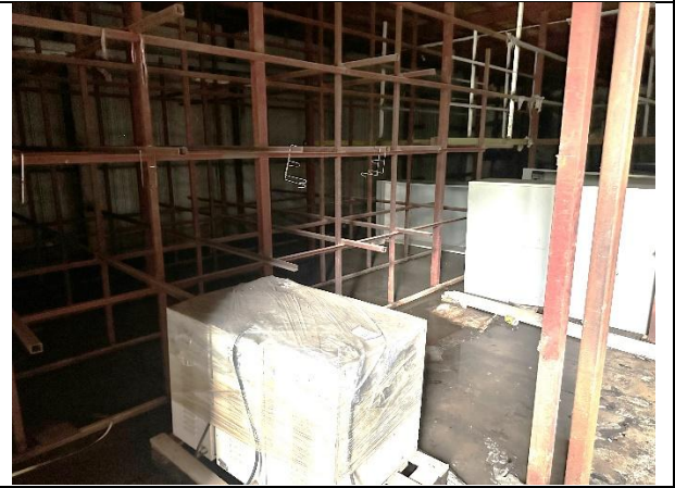
4. Inside the warehouse.
