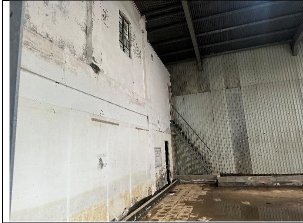
7. Inside the warehouse.
