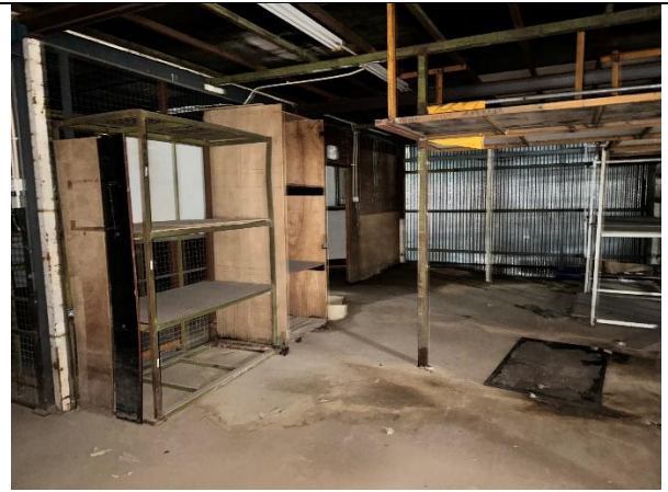
12. Inside the warehouse.
