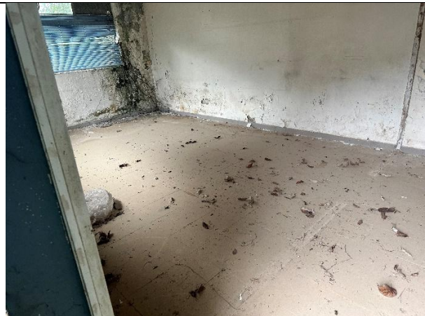
18. Inside the warehouse.
