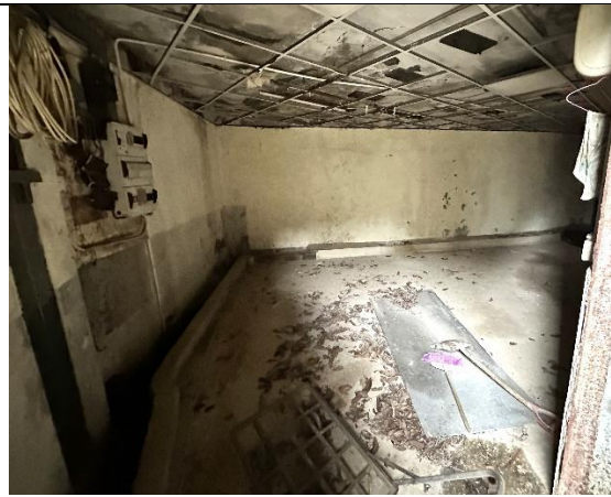
16. Inside the warehouse.
