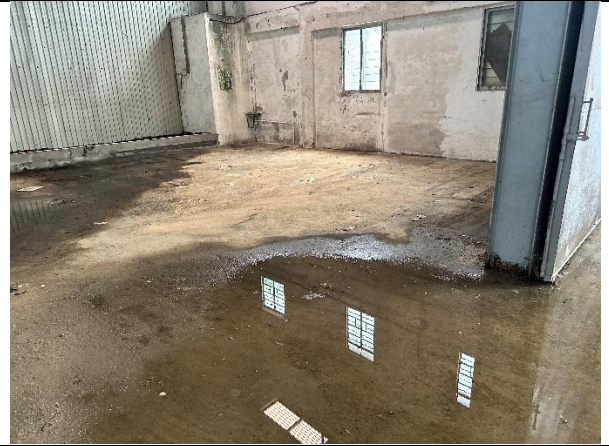
8. Inside the warehouse.
