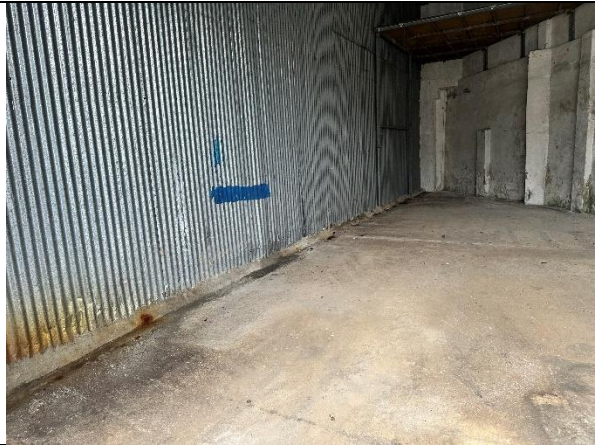
5. Inside the warehouse.
