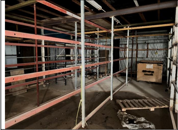
13. Inside the warehouse.
