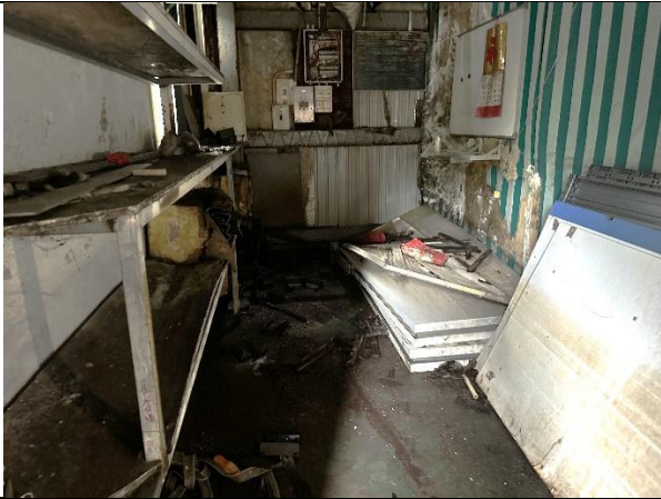
3. Inside the warehouse.
