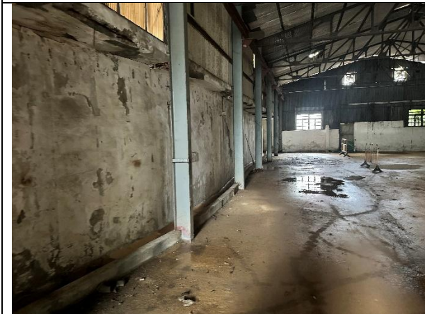
17. Inside the warehouse.
