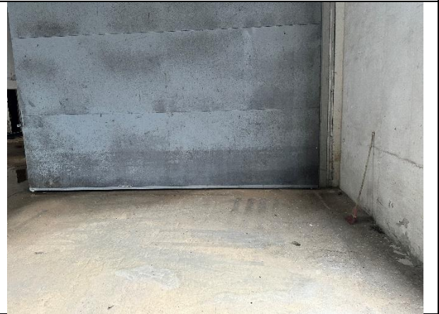
6. Inside the warehouse.
