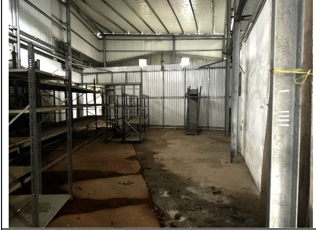
25. Inside temporary structure.
